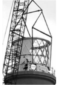
photo BBC: Lifting off the lantern room
